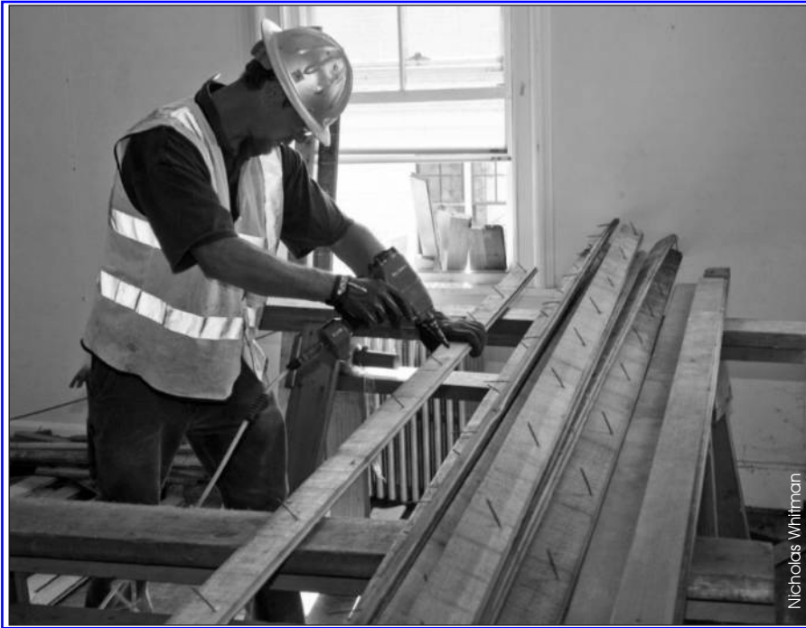
A worker prepares wood for recycling.
